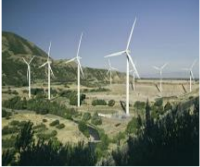
ITD 21 MW – Wind Mill Generators
