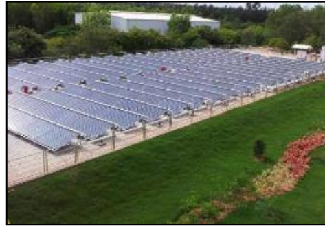
21 KLD heater for boiler water feed
